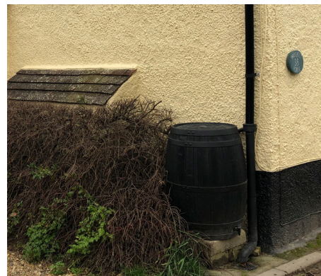
Figure 42: Examples of tanks used for rainwater harvesting
