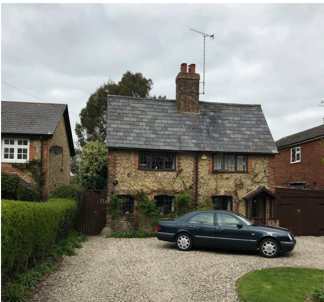
Figure 44: Example of detached housing in Angel Green
