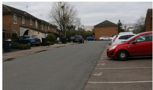
Figure 48: Parking Court on Windmills
