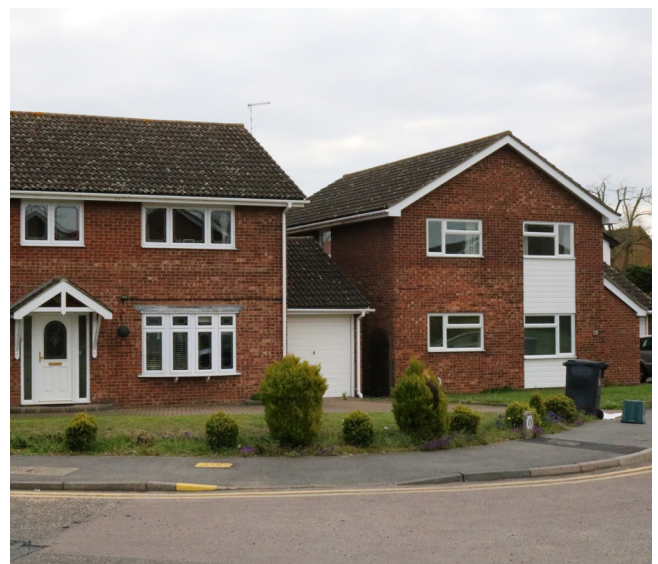
Figure 37: A clear distinction between the road and the property
