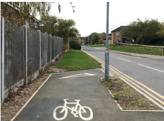
Figure 24: Cycle route on Hospital Approach Road
