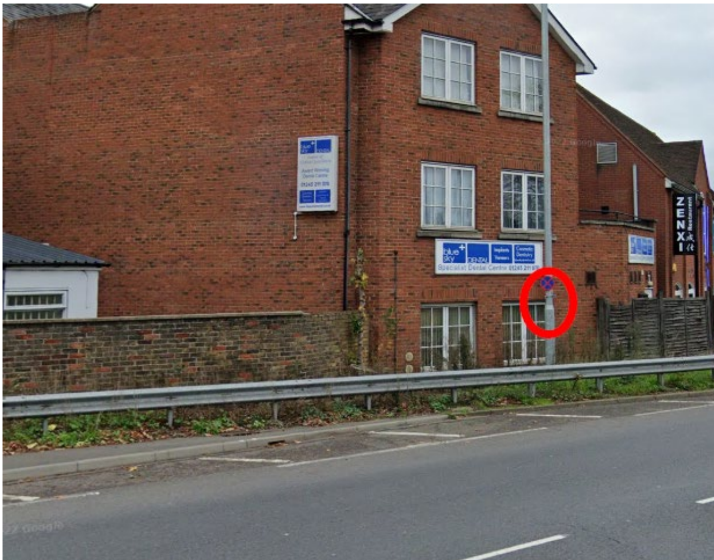
Figure 3.2 - CB98A / CB98B / CB98C Rear of 66 Baddow Road Photograph
