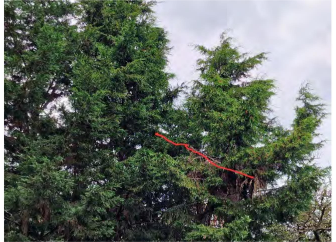
Photo 18. Leyland cypress TG11. The top of one tree has failed and is 'hung-up' over the site. This should be removed.
