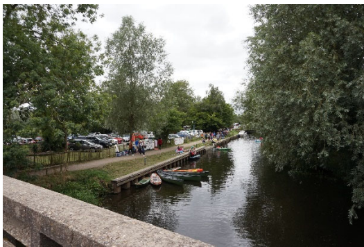
Figure 21 View of Paper Mill Lock from the road bridge
