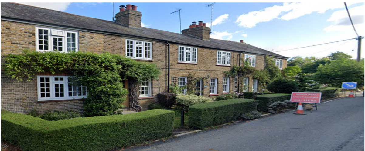
Figure 13. A row of cottages adjacent to St. Mary's Church on Church Road, a fairly unique housing development in Little Baddow, featuring consistent roofline and design, with small but verdant front gardens.
